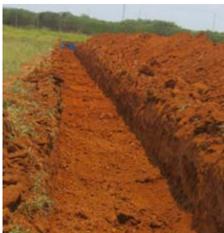
Plate 1. Trenching for runoff collection system.
